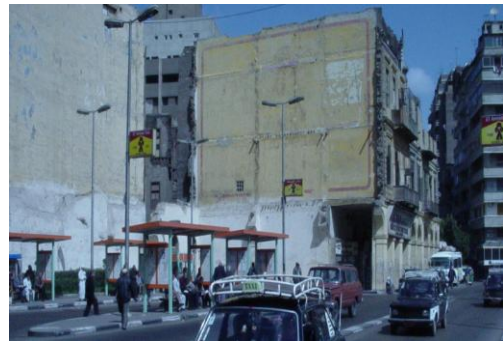
Figure 7 Poorly maintained buildings
